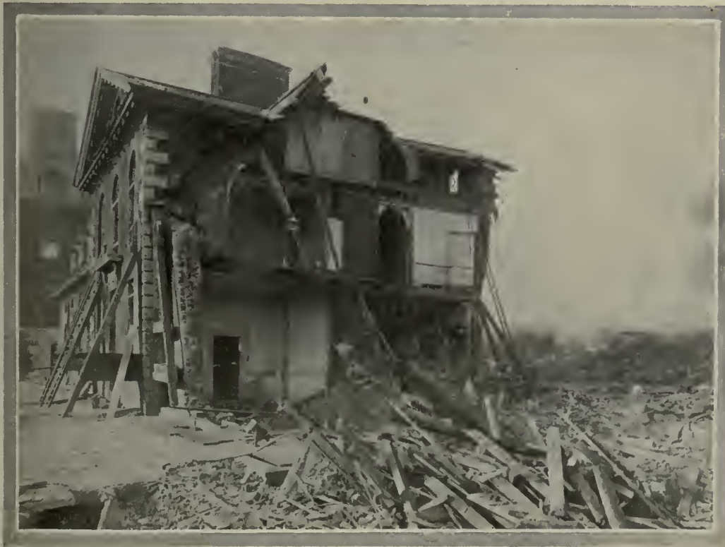
[Official photograph. Crown copyright reserved.]
