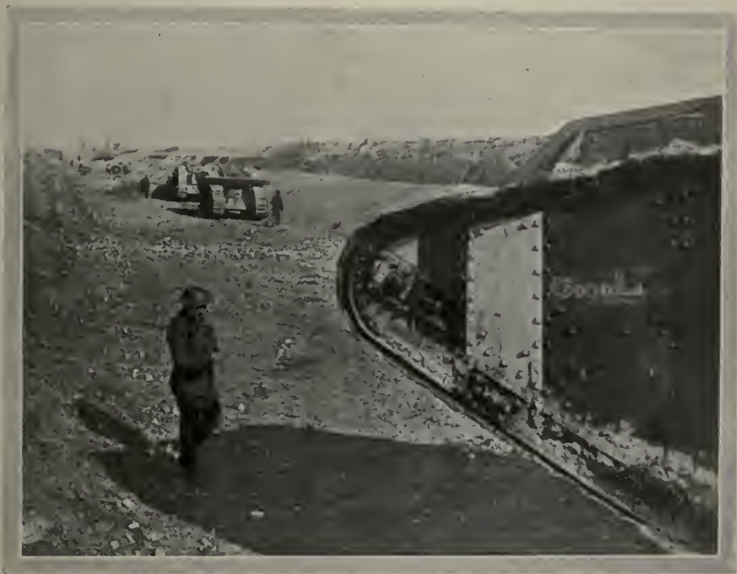
TANKS IN THE CANAL DU NORD.
