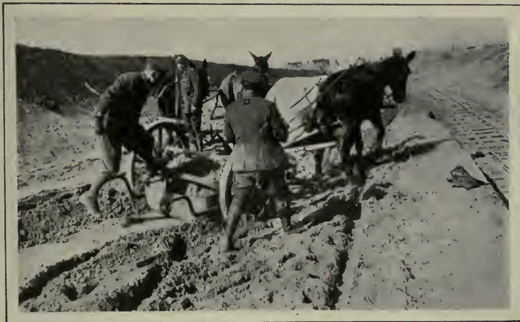
ROAD-MAKING IN THE RECONQUERED AREA: THE SCOPER AT WORK.
