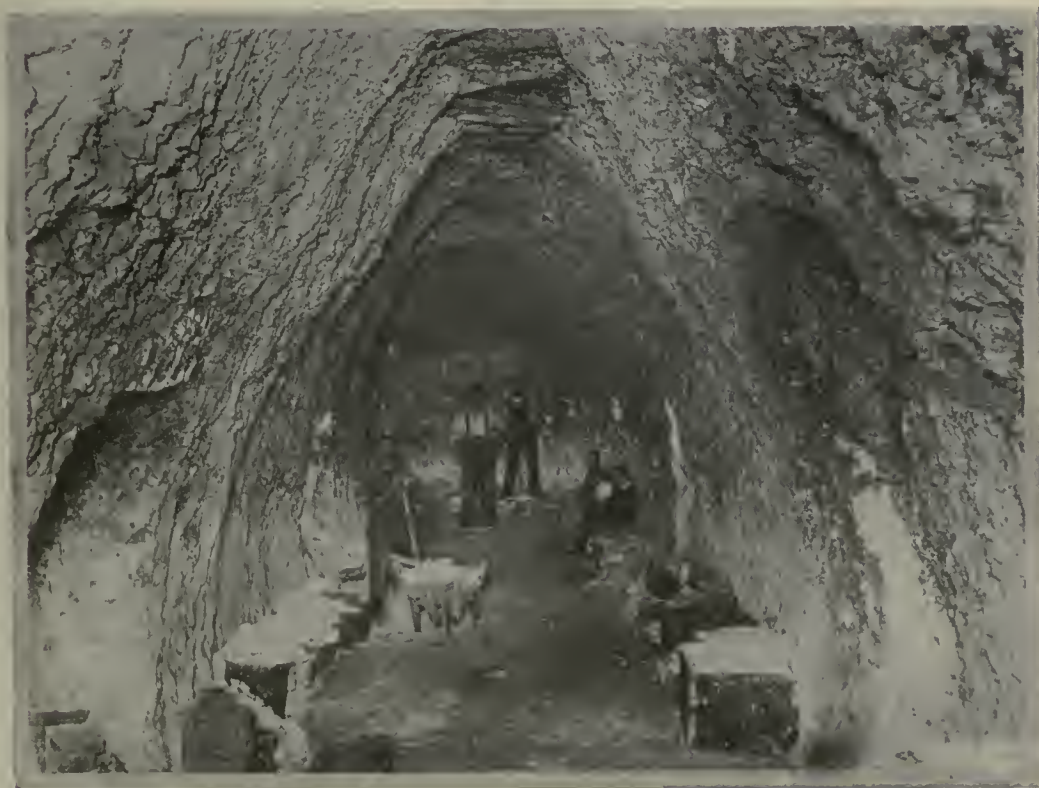
UNDERGROUND SHELTER IN THE CHALK AT RAMSGATE.
