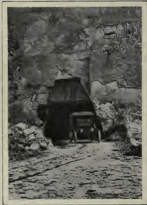
DUG-OUT IN A QUARRY ON THE MARNE.
